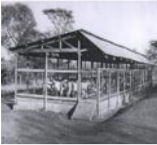
Fig. 40b: Stilted house, slatted floor 30mx5m can hold 300 adult goats
